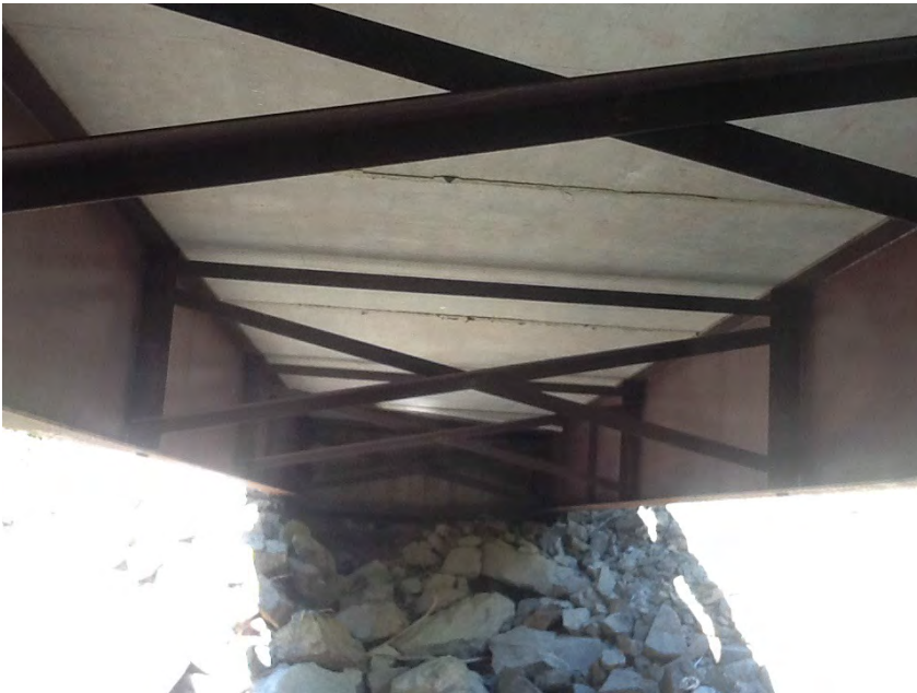
Underside of bridge
