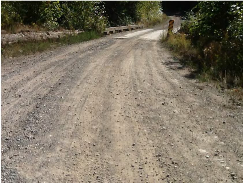
Right approach facing structure
