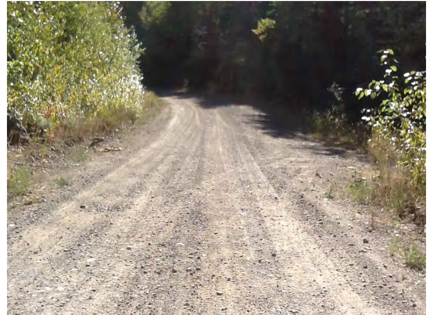
Left approach facing away from structure
