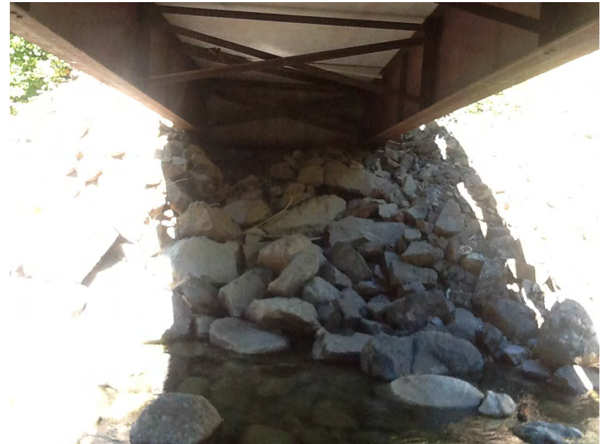
Right Bank Abutment when facing downstream
