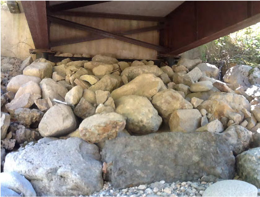
Left Bank Abutment when facing downstream
