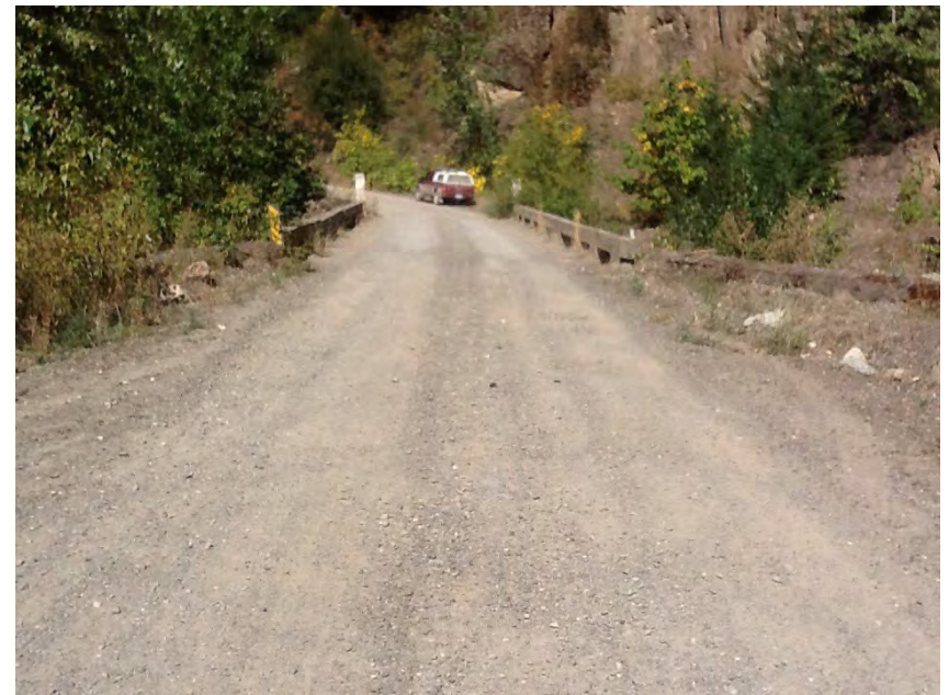
Right approach facing structure
